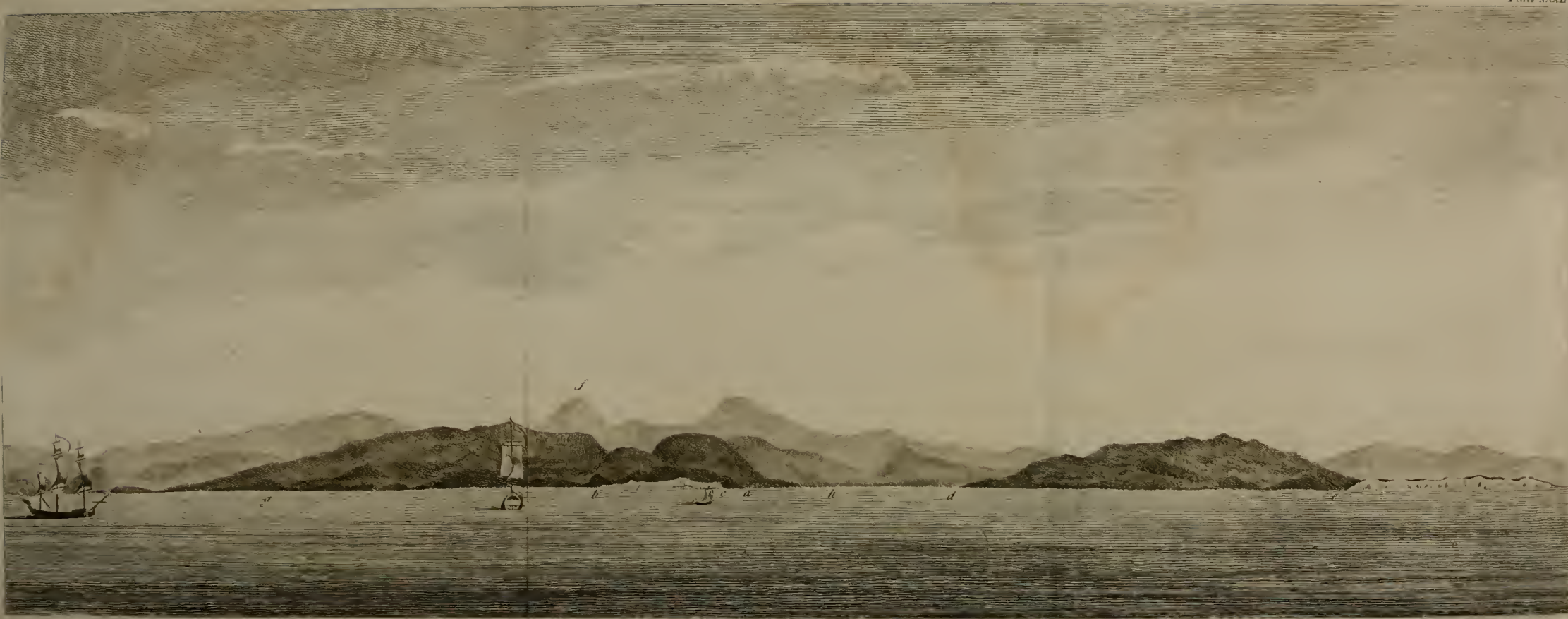
A View of the Entrance of the Port of ACAPULCO.
